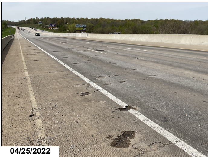
View of spalls in span #2 spalls
