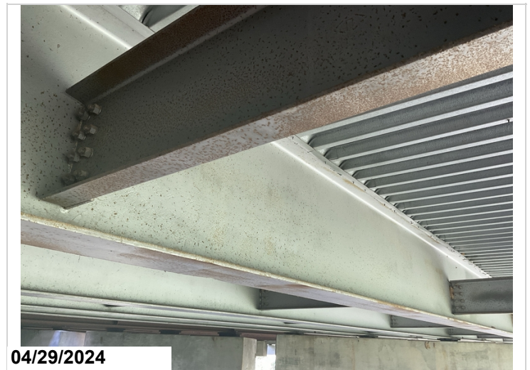
Typical painted beam coating condition.
