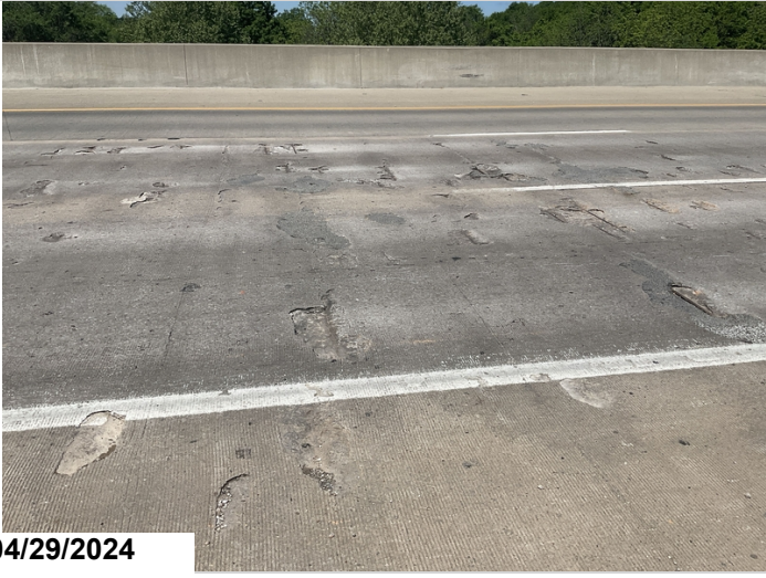
Span #2 delamination
