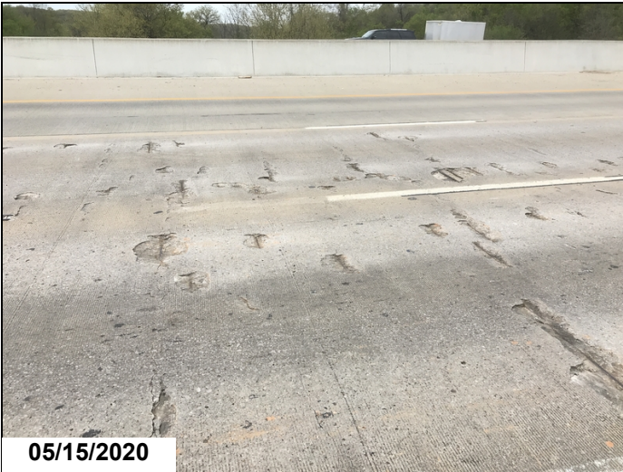
Span #2 middle and right lane numerous spalls with steel exposed.
