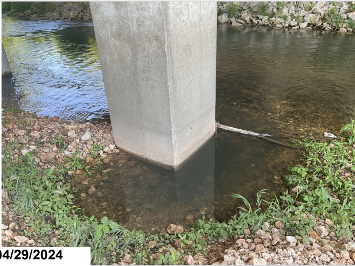
Column #2 of bent #2 is showing cs2 abrasion.
