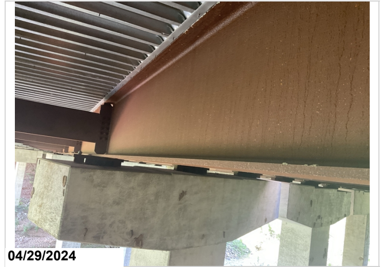
Weathering steel beam condition.
