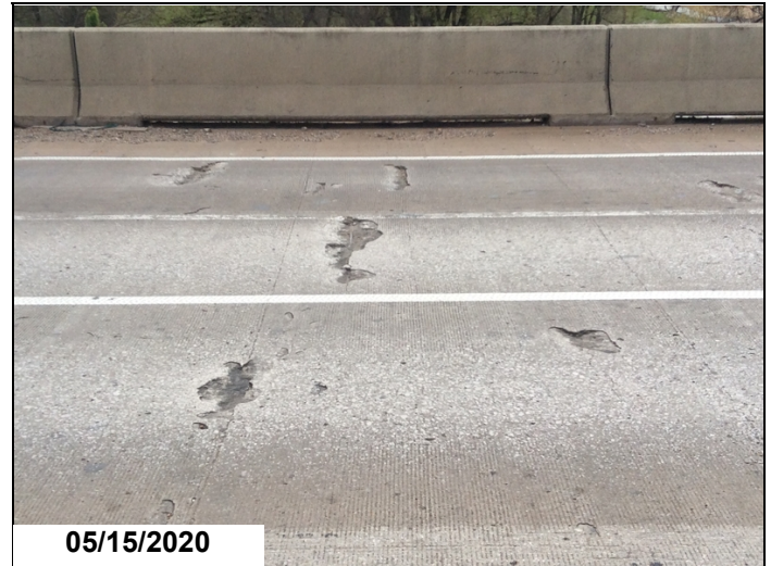
Deck span 2 - scattered deep spalls with steel exposed.
