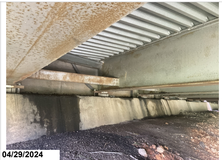
Typical beam corrosion at the beginning of span #1.
