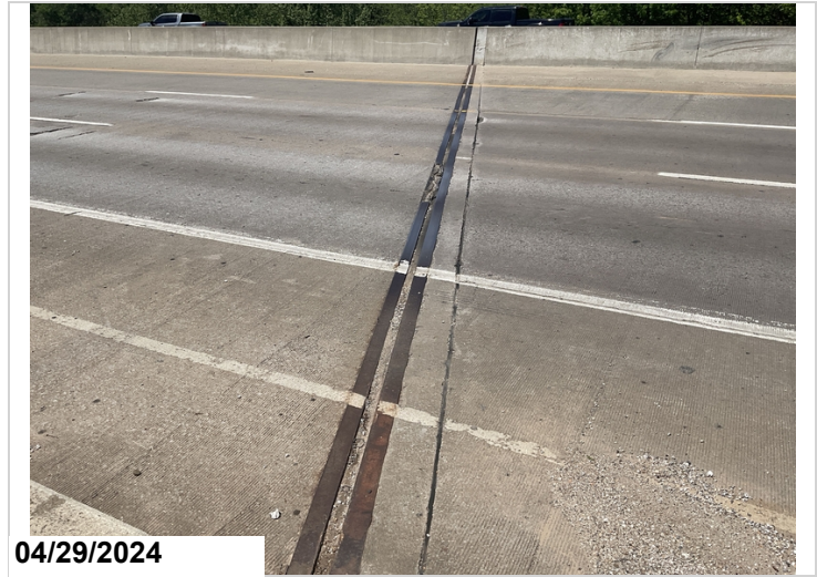
Abutment #2 seal condition.
