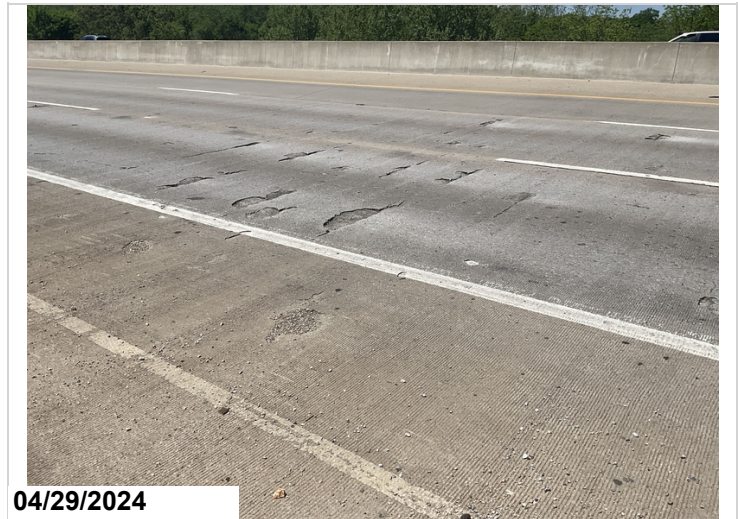
Span #4 delamination
